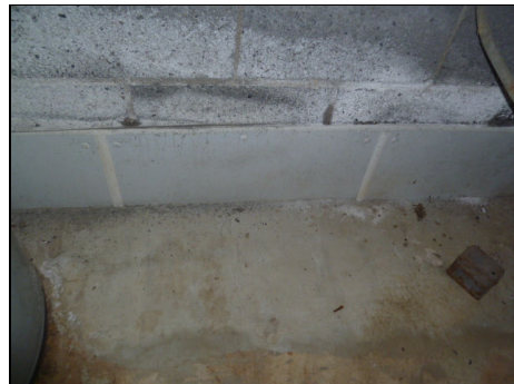
Efflorescence observed at areas of block.
