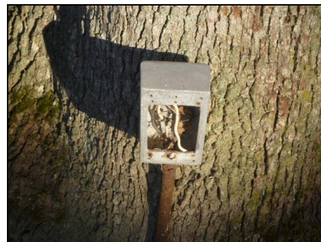
Damaged and exposed wiring at front yard.
