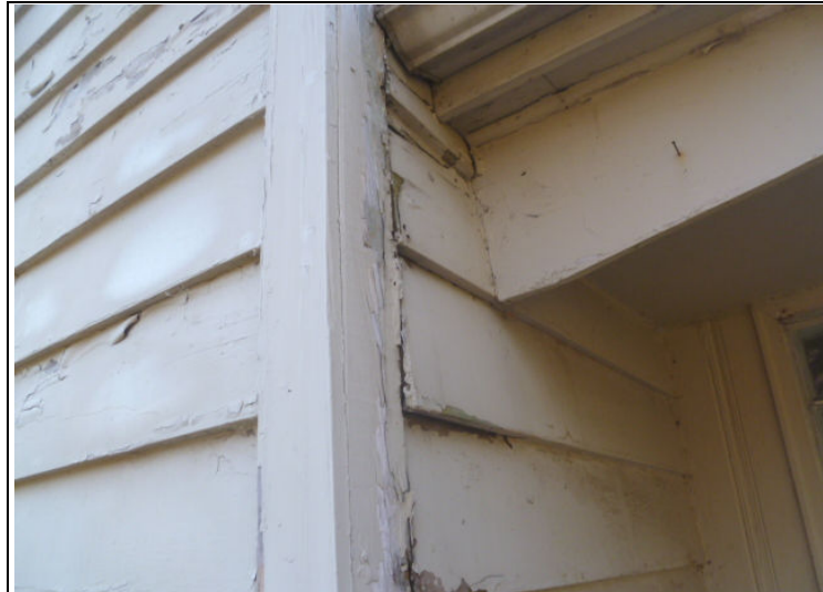
View of water damaged exterior wall materials.
