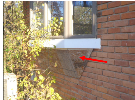
Exposed wood at rear bay window.
