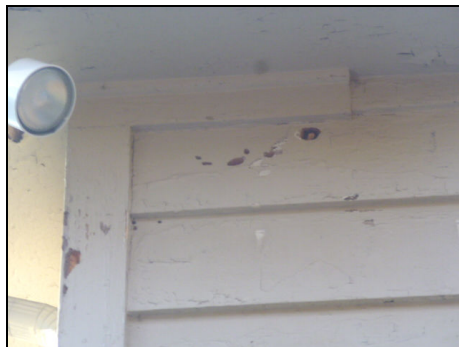
Evidence of wood boring insect damage.
