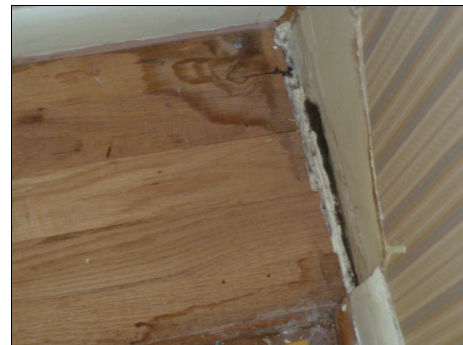
Water staining on floor from exterior leak.
