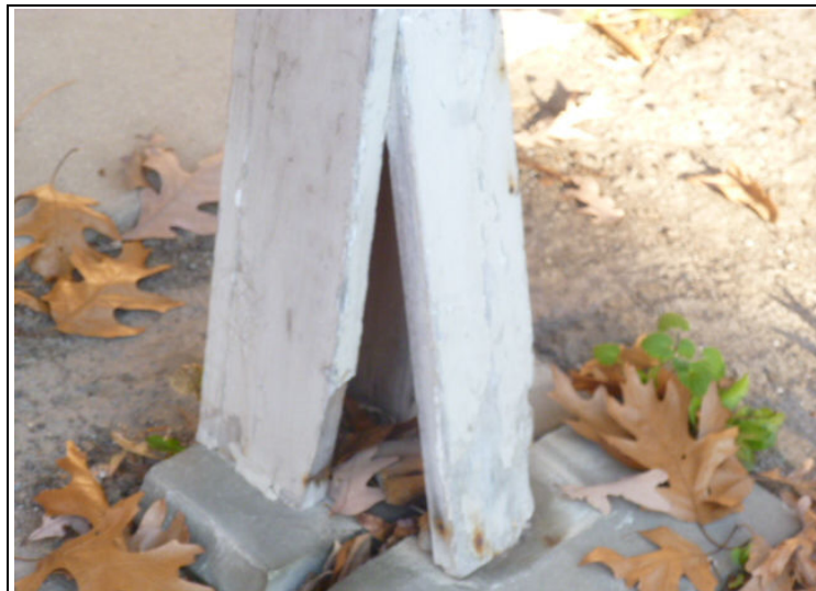
View of damaged support posts serving carport structure.
