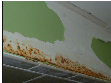
Water staining in bathroom.
