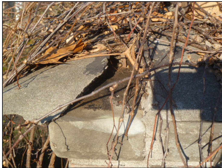
Cap damage on side chimney.
