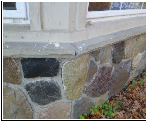
View of loose mortar at stone siding.
