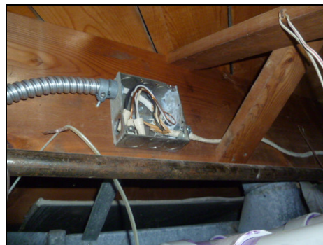
Open junction boxes need to be covered.
