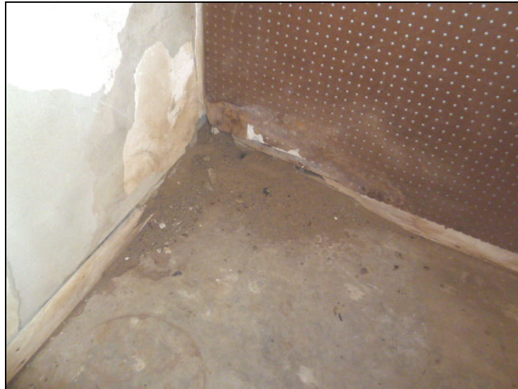
Active leak into garage from exterior wall.
