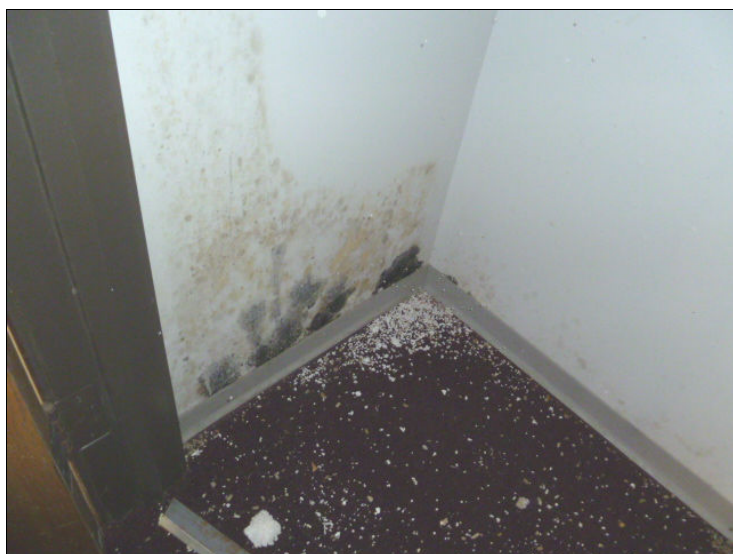
Mold growth within basement drywall.
